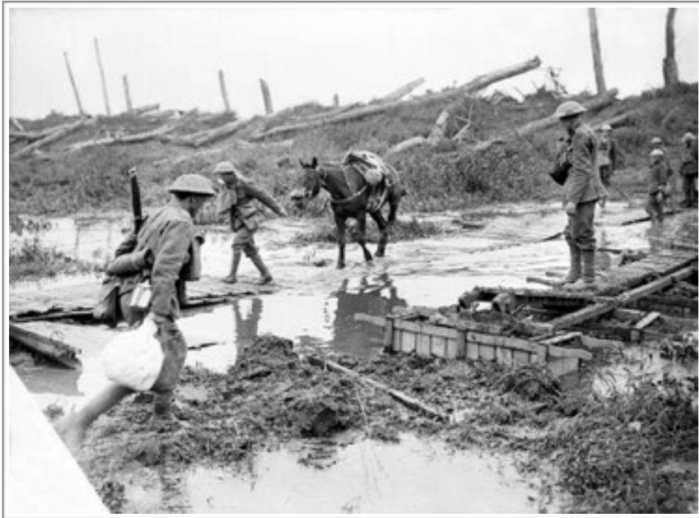
A temporary crossing over the Ypres Canal
