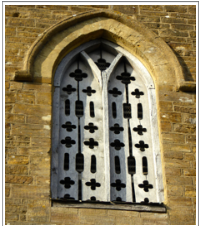
One of the pierced elm screens fitted to the bell chamber openings of Holy Trinity Church, made by John Palmer Rodford in 1919 when he was 70
